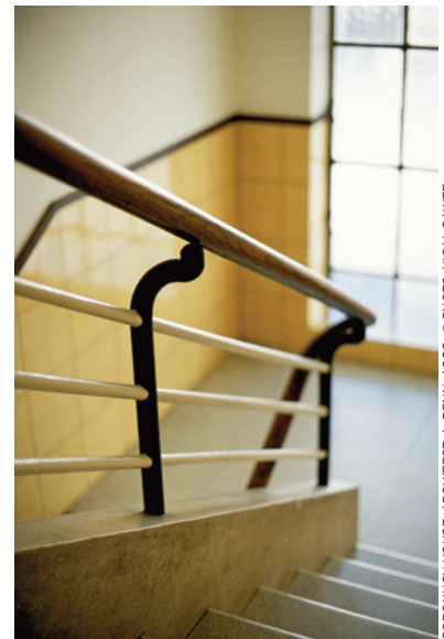
GOROKHOV HOUSE, ARCHITECT: A. PENN, 1938. © PHOTO: YIGAL GAWZE
